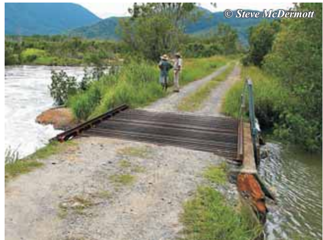
Tidal water entering East Trinity Reserve through a gate in the bund wall during rehabilitation of the area
