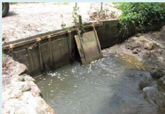
Figure 7. Floodgate on Yorkey's Creek.
